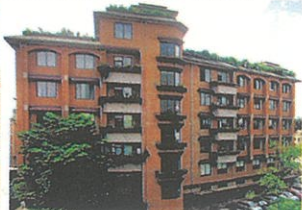
HOTEL OASIS COMMERCIAL BUILDING COMPLEX Patan Dhoka, Lalitpur
