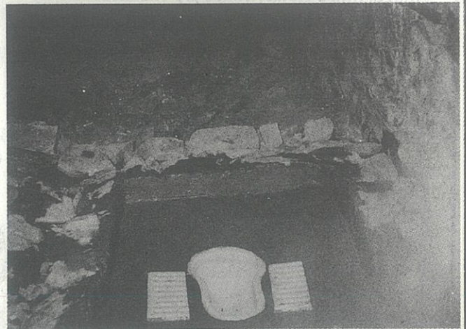
A typical latrine construction with glazed pan provided by project
