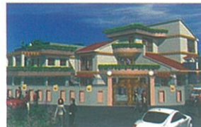
RESIDENTIAL BUILDING OF Rtn. B.L. Mallapaty Location : Bhainsepati, Lalitpur
