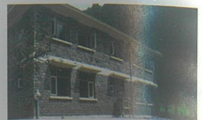
JIRI HOSPITAL REHABILITATION PROJECT OT/IPD BLOCK Location : Jiri, Dolakha
