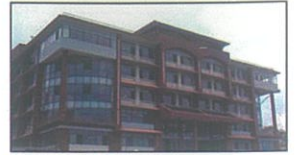
View of building from Kantipath
