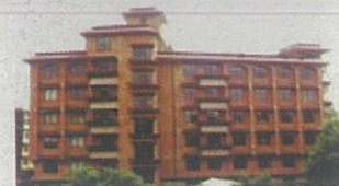
NEPAL BAYERN ELECTRIC BUILDING COMPLEX Patan Dhoka, Lalitpur
