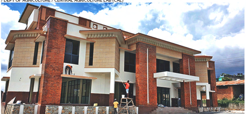
JAWALAKHEL HANDICRAFT CENTER / JHC Building (Nearing Completion)
