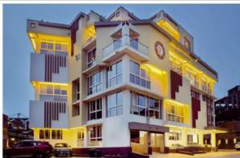
HIMALAYAN BANK BRANCH OFFICE BUILDING, DURBAR MARG
