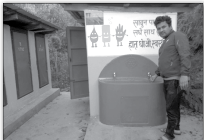
Upgrading of WASH Facilities in School in Mirge Village Dolakha under GG1641893.
